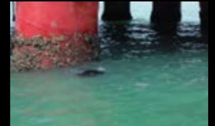
Offshore Infrastructure Inspections
