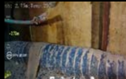
Outer Pipeline Inspections
