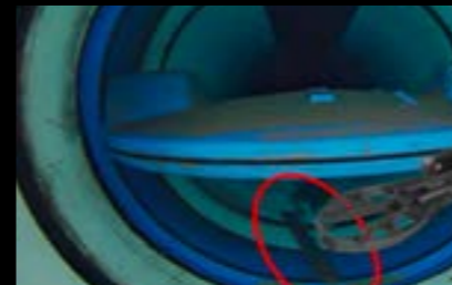
Pipeline Valve Inspections
