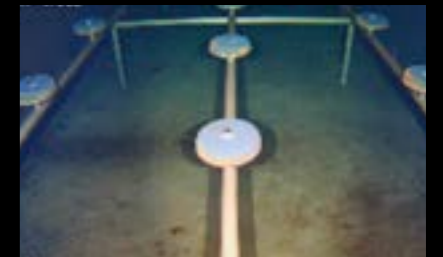
Aeration Disc Inspections
