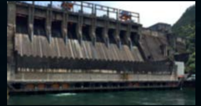
Inspection at China's Xin'anjiang Hydropower Station
