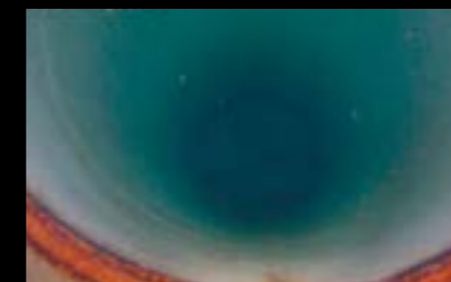
Supply Pipe Inspections
