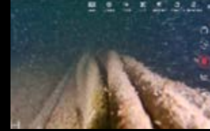
Pipeline Inspection & Maintenance
