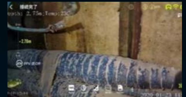
Underwater pipeline inspections conducted in Japan
