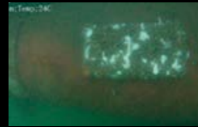
Sacrificial Anode Inspection & Cleaning
