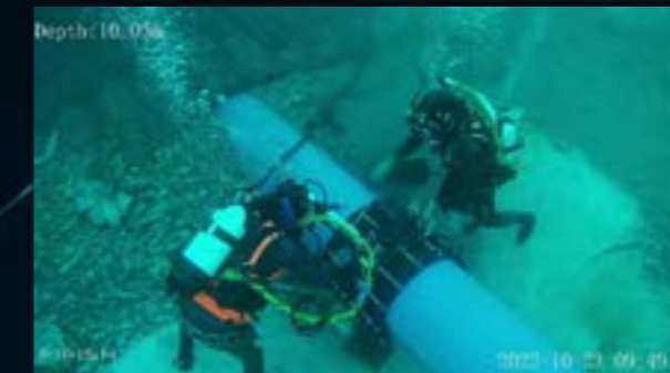
Underwater pipeline maintenance and monitoring for damaged pipelines in Greece
