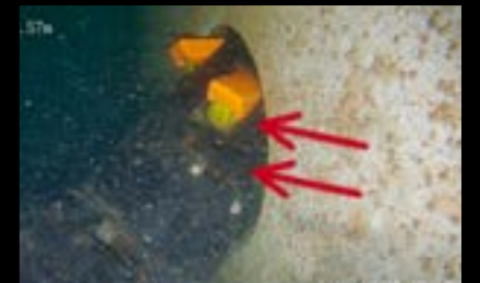
Bend Restrictor Inspections
